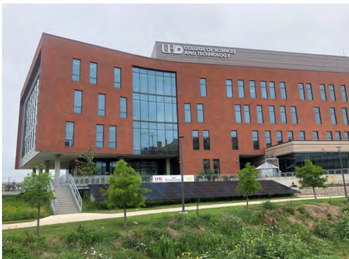
Science and Technology Building. Read more about the recently installed solar panels in Vol. 66, Iss. 1. Photo credit: Shaheryar Khan.
